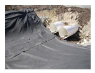
**ABMAT**<sup>™</sup> Geo-Fabric is constructed of needle punched Polyester short filaments. These filiments form a stable matrix exhibiting excellent strength and hydraulic characteristics. Allowing this product to be used for numerous situations where an economical solution is required for filtration and soil stabilisation in domestic landscaping applications.
